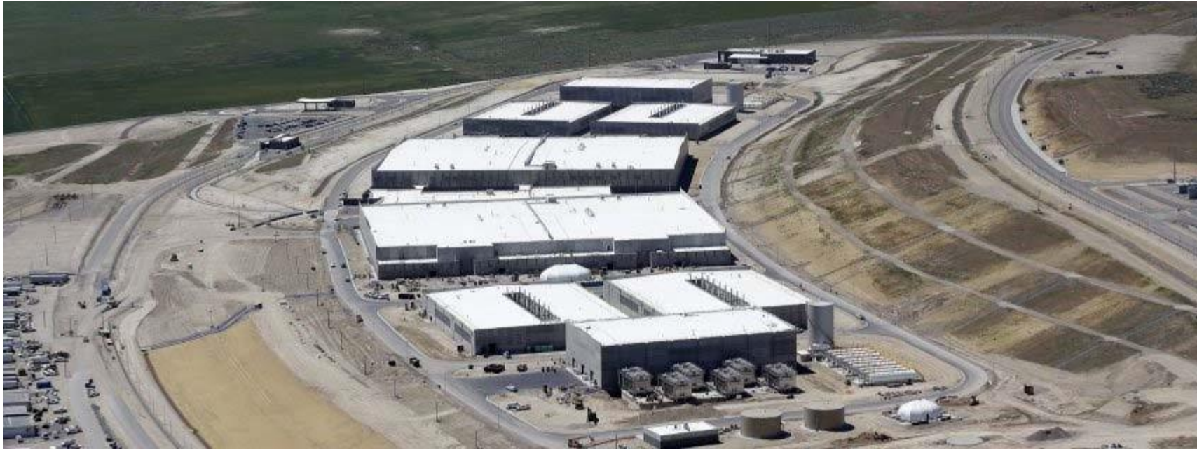
NSA data center Utah – 3 \times 10^{18} - 10^{24} bytes
