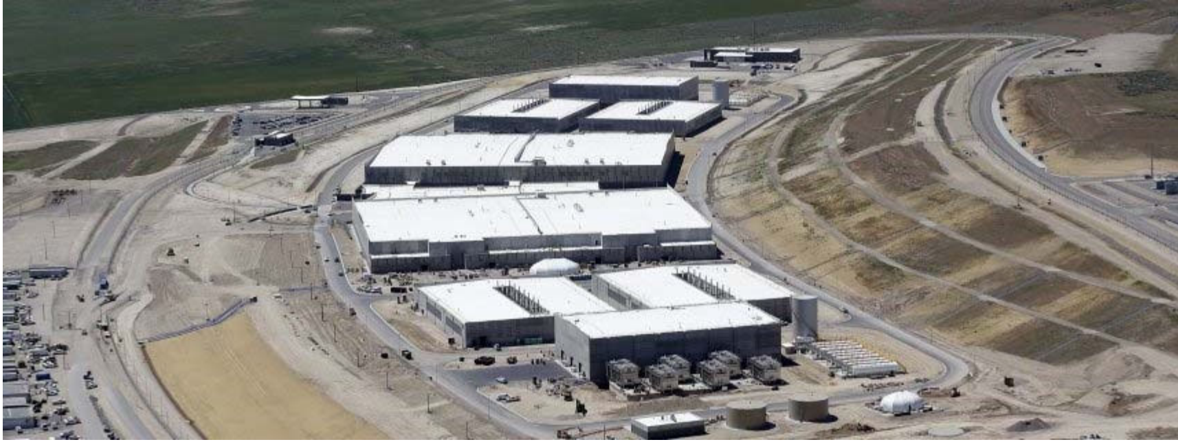
NSA data center Utah – 3 \times 10^{18} - 10^{24} bytes
